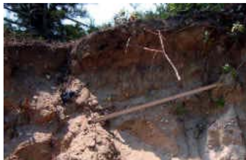
Figure 5 - Till draping hill of outwash material at East Moriches Retirement Village. South is to the left of figure. Stick is one meter in length.
